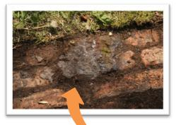
On the brick floor, there is still evidence of pitch used to waterproof boat hulls – it dripped down and set solid on the floor.
